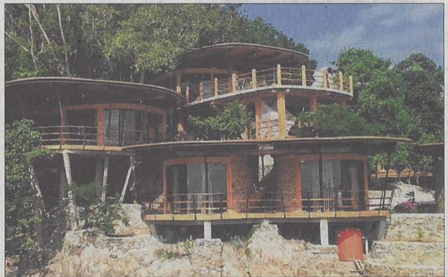
The air-conditioning systems of the new villas will be powered by blocks of ice which are frozen in the day using solar power. PHOTO: LOOLA ADVENTURE GROUP
